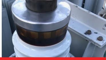
Belzona 9611 (ES-Metal) and Belzona 1161 (Super UW-Metal) were used to repair the equipment. Belzona 9611 (ES-Metal) is a rapid curing putty grade system which is ideal for sealing low pressure live leaks prior to application of additional Belzona systems to create a more permanent repair.
