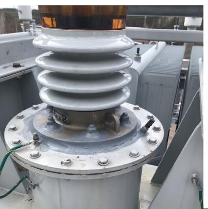
Belzona 1161 (Super UW-Metal) was then applied in conjunction with Belzona 9341 (Reinforcement Tape) around the bushing to provide a more permanent repair. The bolts of the bottom flange were also sealed.
