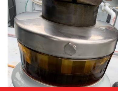
A transformer station in Northwestern Ontario, was having issues with the bushing of a transformer that was leaking oil. The leaks were causing an environmental hazard as well as the inconvenience of having to top up the oil in the transformer every couple weeks. There was no way of sealing these leaks, welding was not an option due to the environment.
